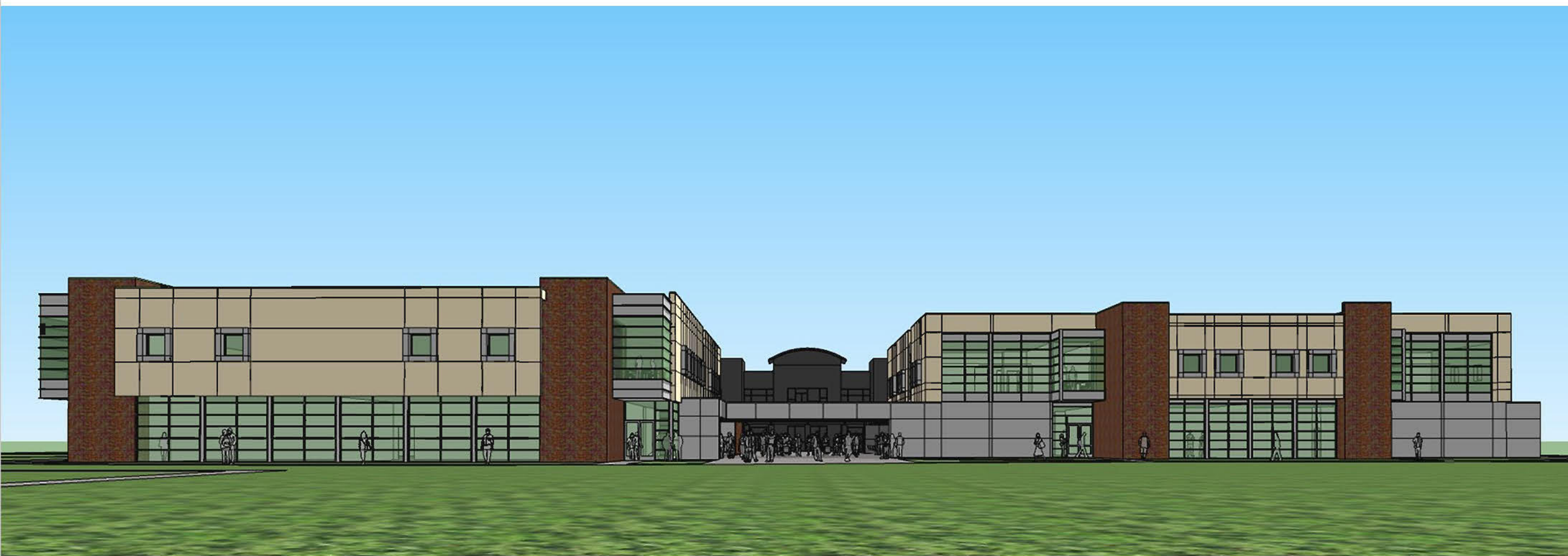
BOTH BUILDINGS VIEWED FROM PECAN BOULEVARD
